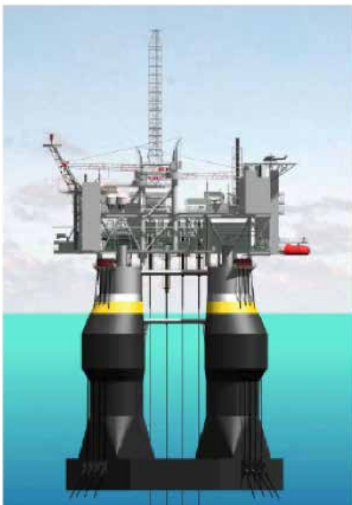
FIG 12: SMALL, FLOATING, INTERVENTION, PRODUCTION, OFFLOADING SYSTEM WITH DRY-TREE PREDRILLED WELLS
