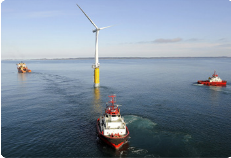
The first pilot wind turbine of the Hywind concept was deployed southwest of Karmøy, Norway, in autumn 2009. Photo: Statoil.
