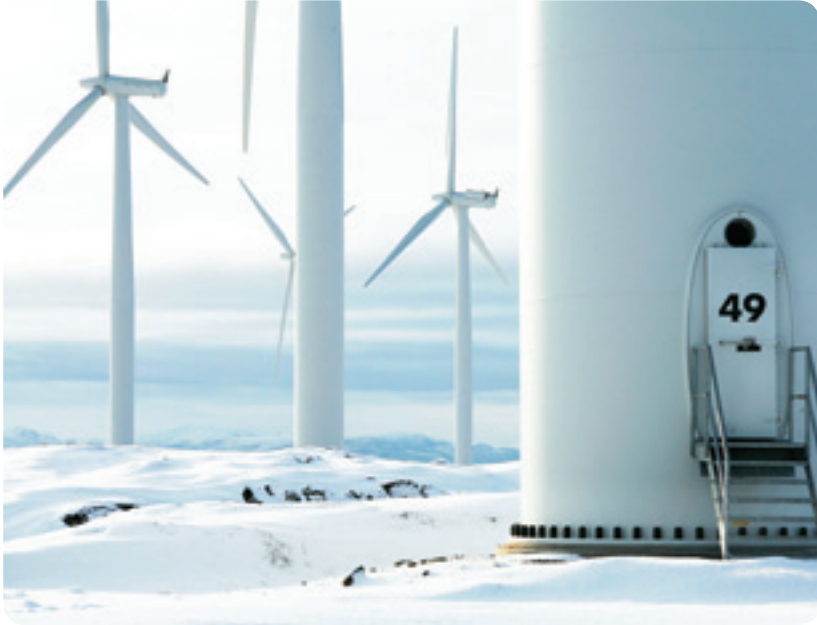
Smøla Wind Farm. Photo: Statkraft.
