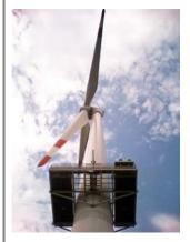
A prototype of Senvion (formerly REpower Systems SE) is operated close to Bremerhaven since 2008. The REpower 5M is an offshore turbine with a capacity of 5 megawatts and was installed on a jacket foundation. This turbine and foundation type were later used for 6 turbines in the alpha ventus offshore test field.
